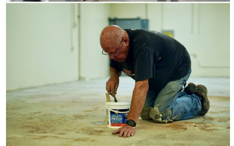
Students and community members prepare the floor for its new epoxy coat.
