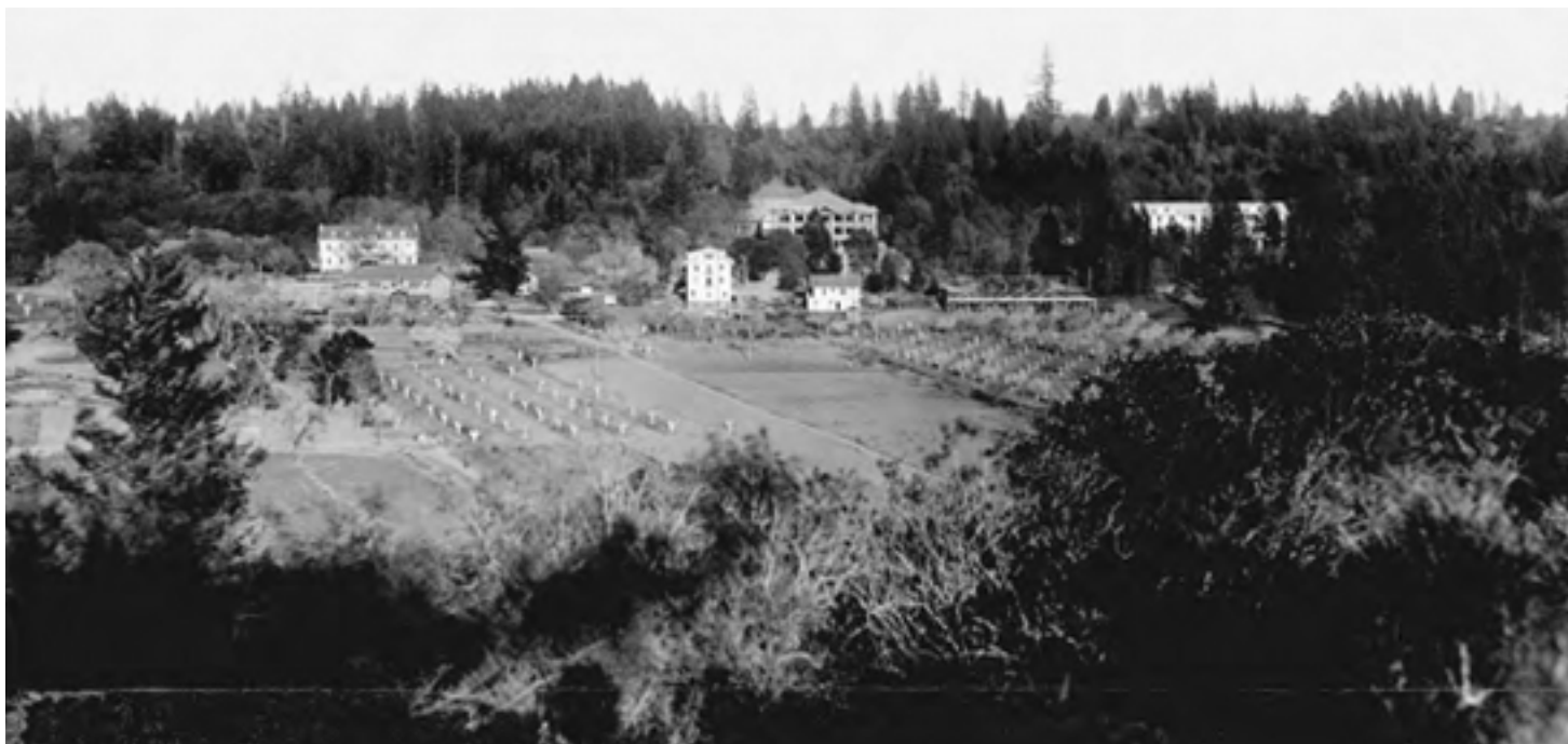
Campus, circa 1919, with Irwin Hall under construction
