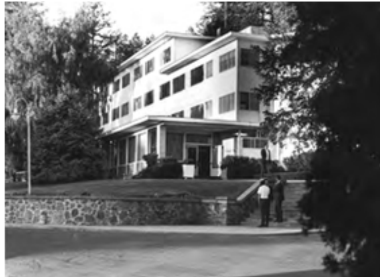
TOP: Construction of Newton Hall, 1951, Grainger Hall in the background; ABOVE: Newton Hall main entrance
