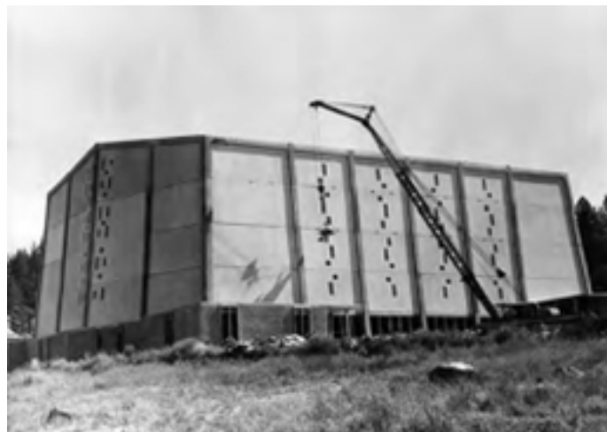
Church Sanctuary under construction, 1967-68
