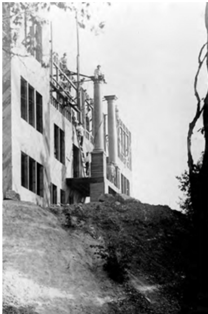
Irwin Hall porch under construction
