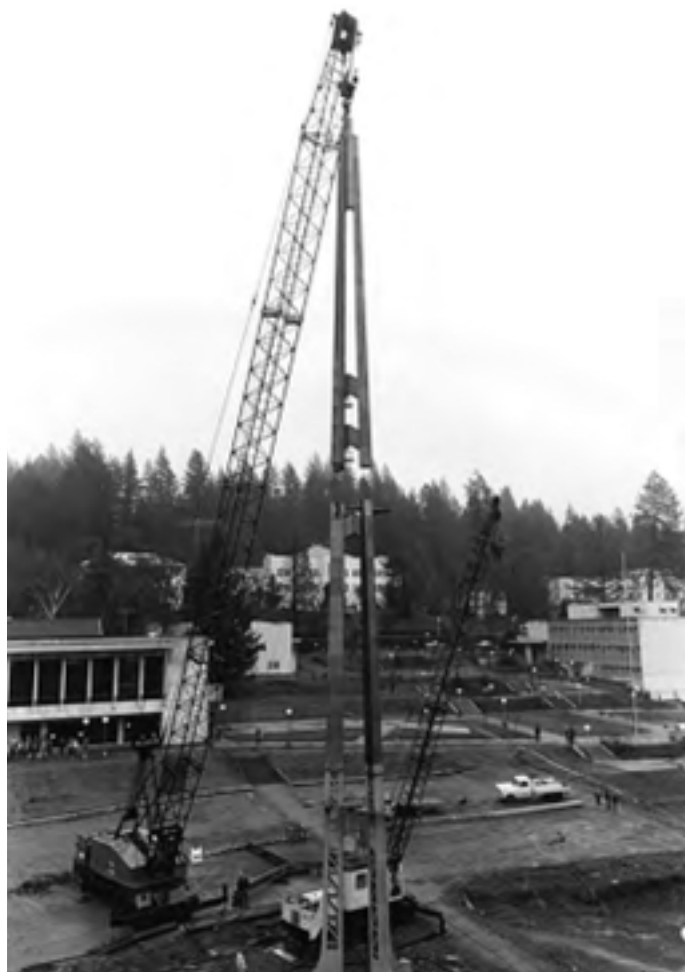
Installation of the bell tower; Dining Commons at left
