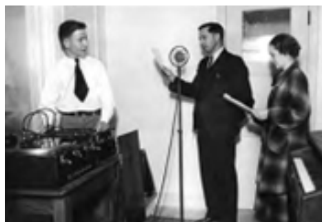
TOP: Milford Nelson operates P.U.C.'s first radio transmitter, West Hall, 1927;
